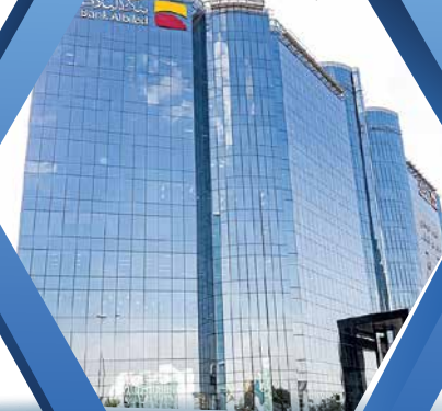
Ksa Alhilad Bank Projesi
